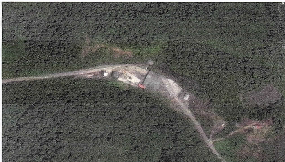
Figure 8 Labu Control Post
