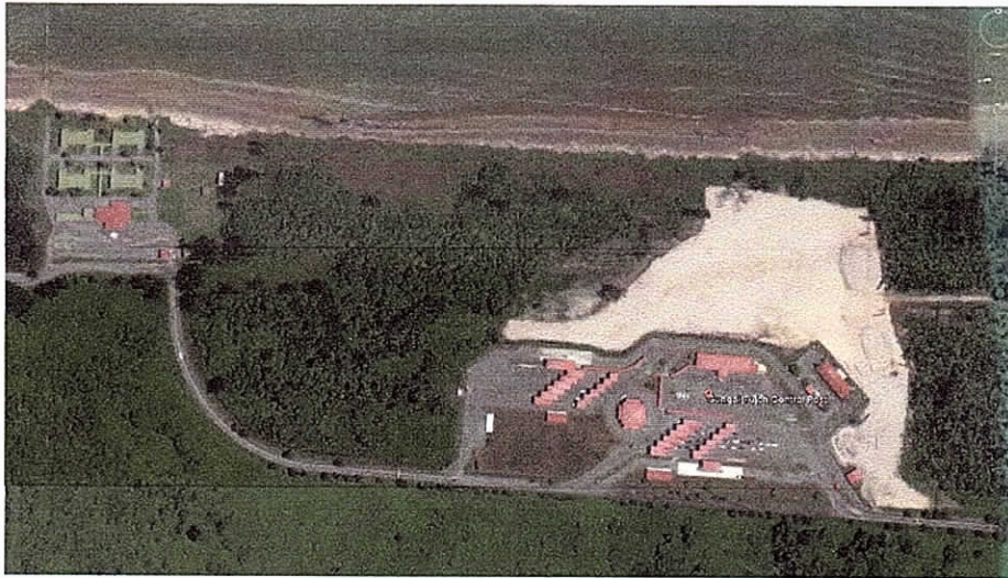
Figure 1 Sungai Tujoh Control Post
