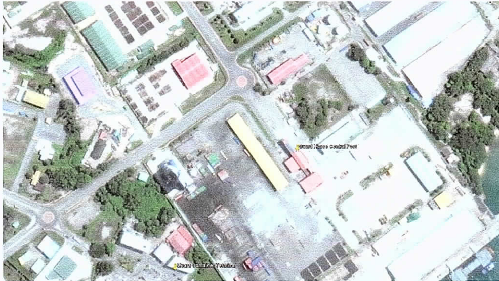
Figure 5 Guard House Control Post
