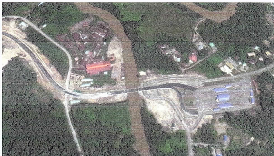
Figure 9 Ujung Jalan Control Post
